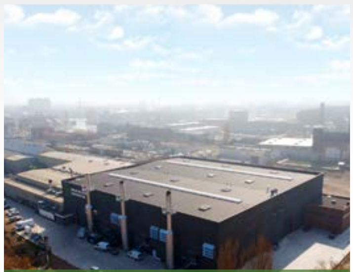
ABC headquarters and production facility in Ghent, Belgium
